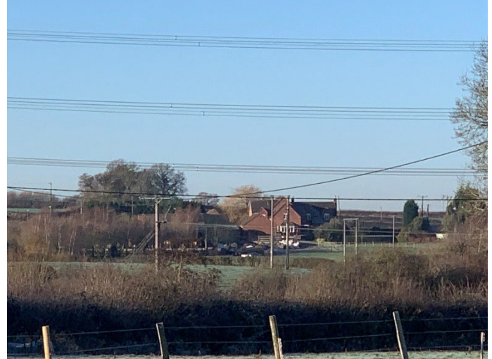
View of the east facing façade, taken from Old Byre (Walton Lane Farm).
