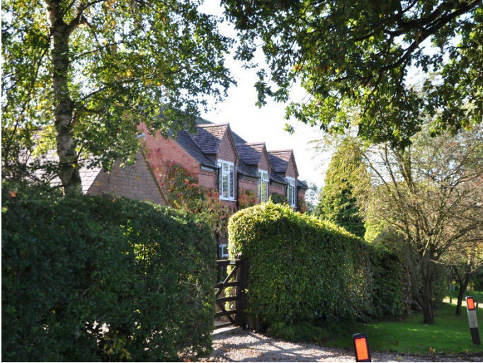
View of the north facing front façade of New Corner Farm (to the left) and Corner Farm (to the right).
