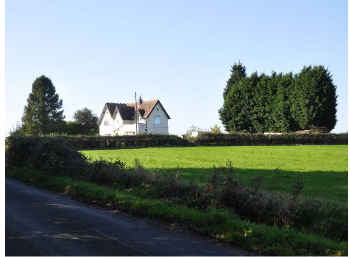
View of property showing eastern façade (to the left) and western façade (to the right).
