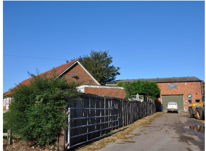
View of No. 3 and 4 Oaklands Farm Cottages with farm buildings to the rear.
